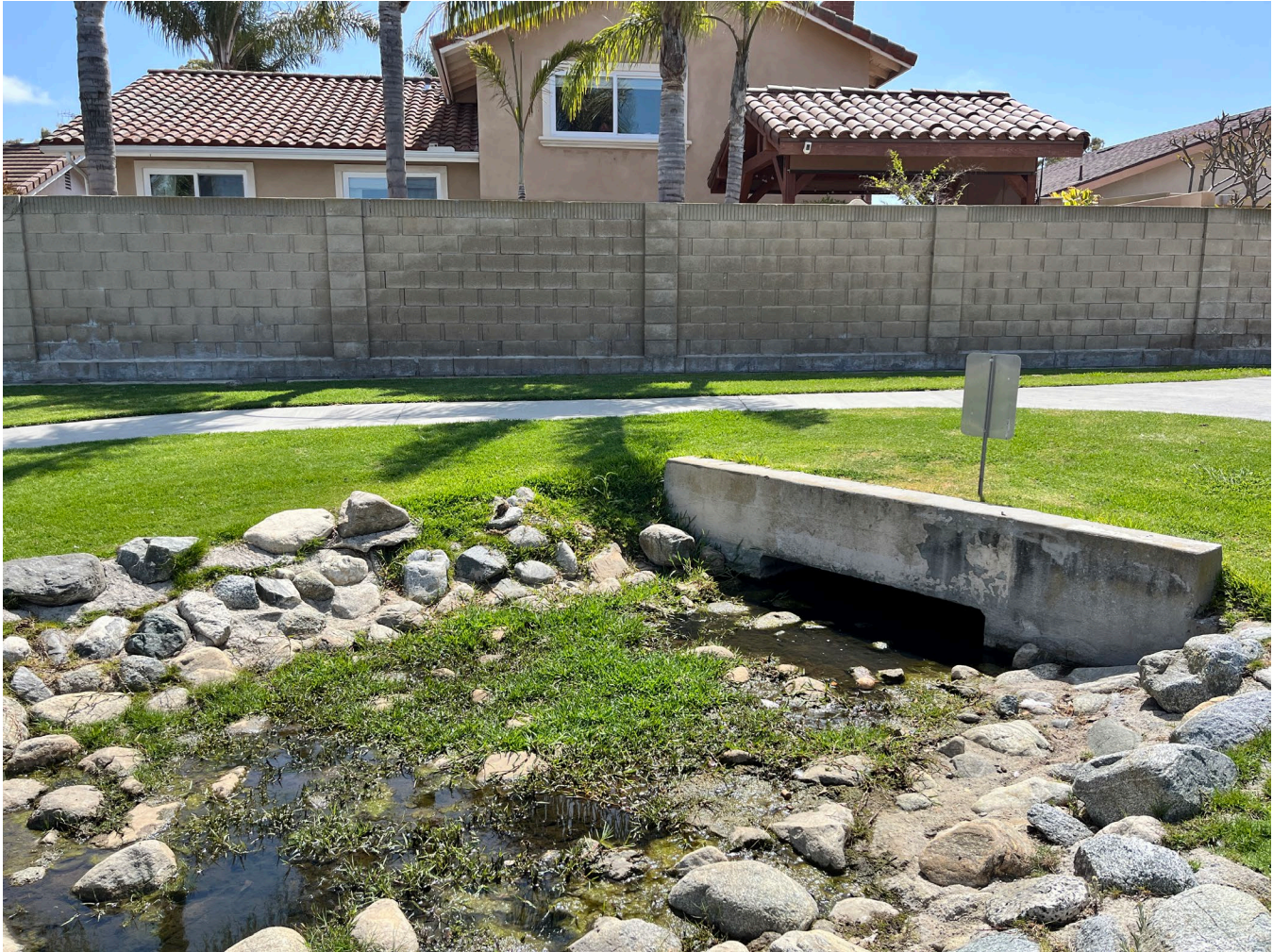
Figure 1-6. Headwall at southeast corner of Greer Park lake.
